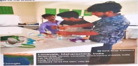
Polythenes ,rapers etc along with sand was filled with the stick to poke the plastic waste inside the bottle down so you can fit as much as possible into it.
